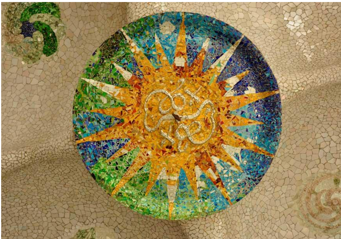
Detail from the roof of The Park Güell Designed by Antoni Gaudi 1906
